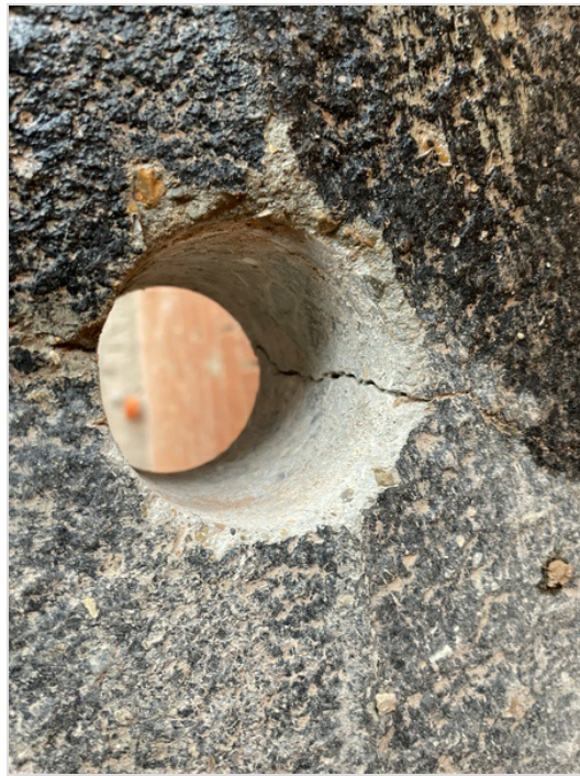
Barst thv boring ~ wapening vrijmaken
